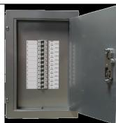
Turn off power 120VAC to the heater. Check your breaker panel and disable the power to the OASIS heating elements.
