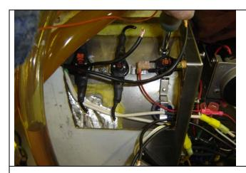
Unscrew the DC high limit aquastat, this will give you access to the AC high limit aquastat mounting
