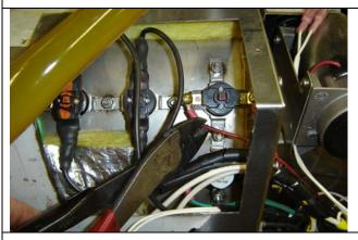
Replacing the DC high limit aquastat. (with screw connectors)
