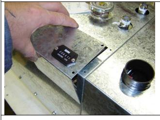
Close aquastat cover. Turn power back on and test operation of the heater.
