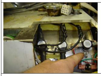
Replacing the DC high limit aquastat. (with tabs)
